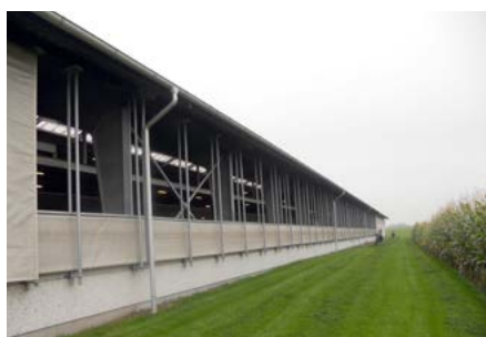
Figure 8. Shows lifting side inlet ventilation
