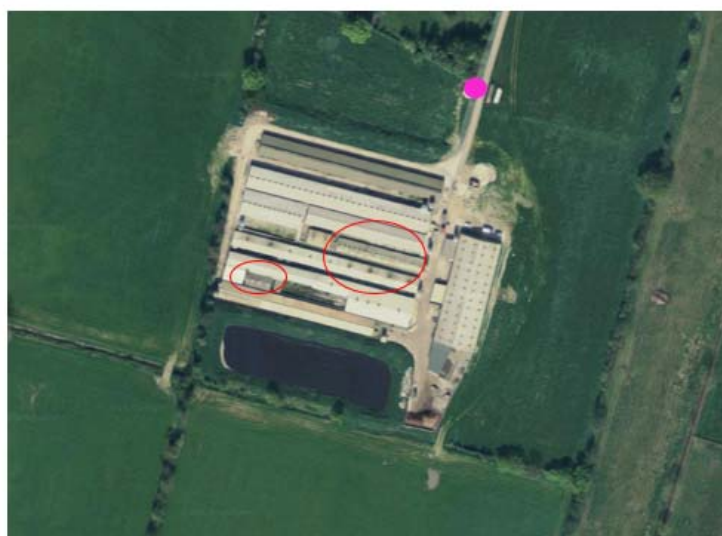
Farm layout: Purple circle = borehole position. Red circle = the two first-stage weaner buildings holding pigs from weaning
