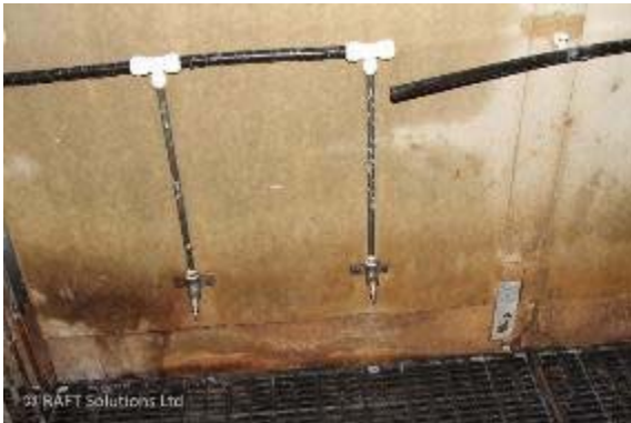
Figure 36. (left) and Figure 37. (right) Contamination found within the pipework demonstrating the presence of biofilm
