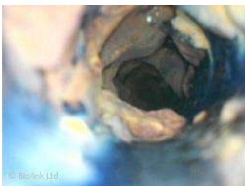
Figure 32. Biofilm lining the inside of a water pipe
