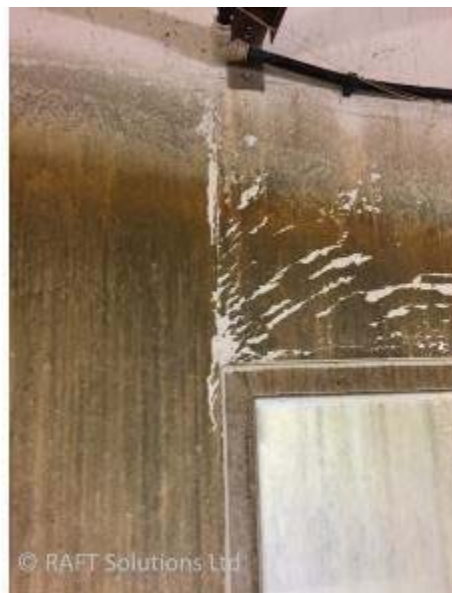
Figure 28. (left) and Figure 29. (right) Evidence of iron (orange) and manganese (black) deposits within limescale deposits left from a piggery sprinkler system
