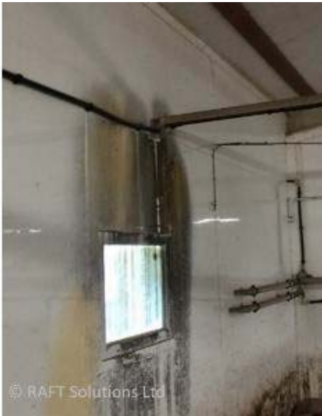
Figure 28. (left) and Figure 29. (right) Evidence of iron (orange) and manganese (black) deposits within limescale deposits left from a piggery sprinkler system
