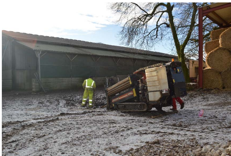
Boring machine placing pipe underneath a building
