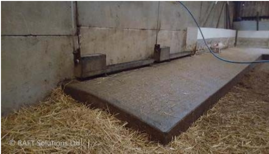
Figure 42. Example of how an angled plinth can help to encourage the correct drinking posture and reduce risk of fouling in the water delivery system
