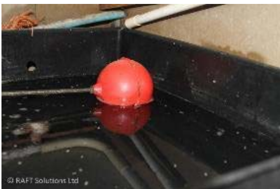
Figure 34. (left) and Figure 35. (right) Biofilm presence in a header tank
